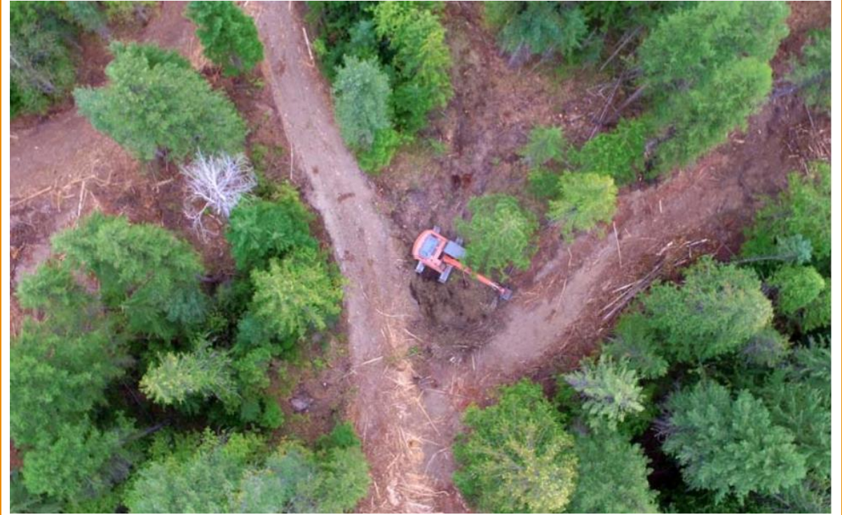
Aerial view of mechanical piling of post-harvest fuel load with excavator
