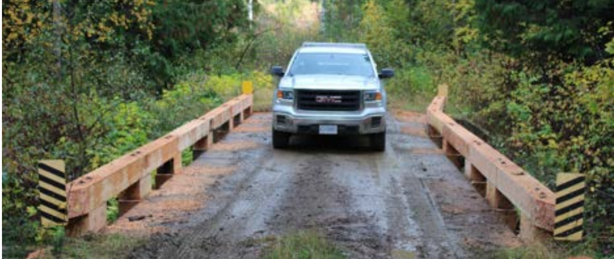
LNTCF SAWMILL CUT TIMBERS FOR BRIDGE REPAIR
